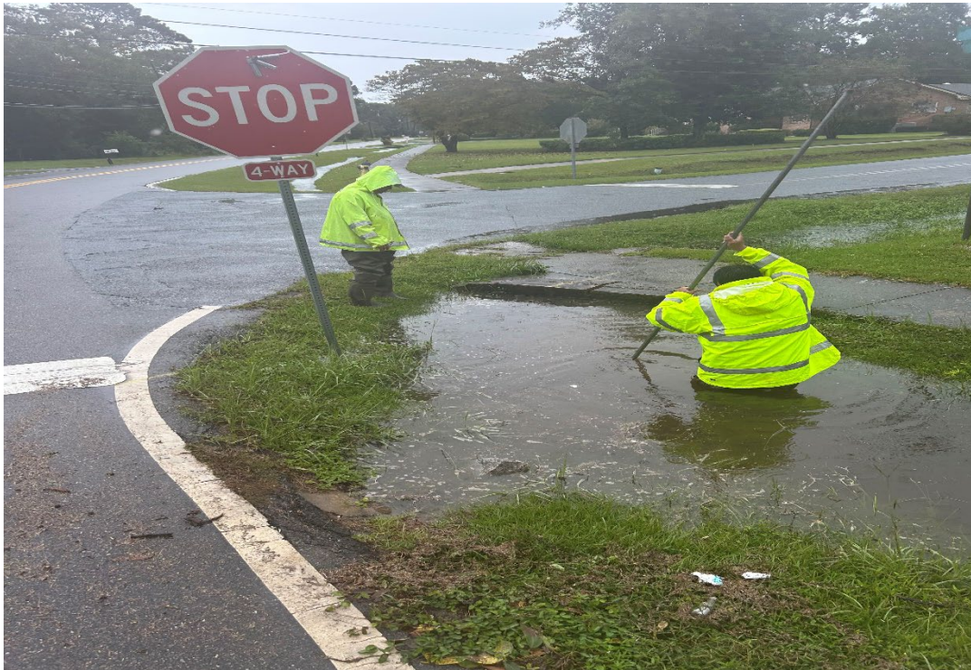
Clearing Culvert at Rommel Ave. September 26, 2024
