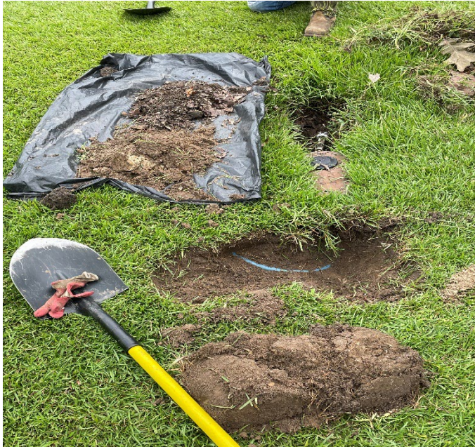
Releasing air for effluent lines. Pipe Makers Canal September 27
