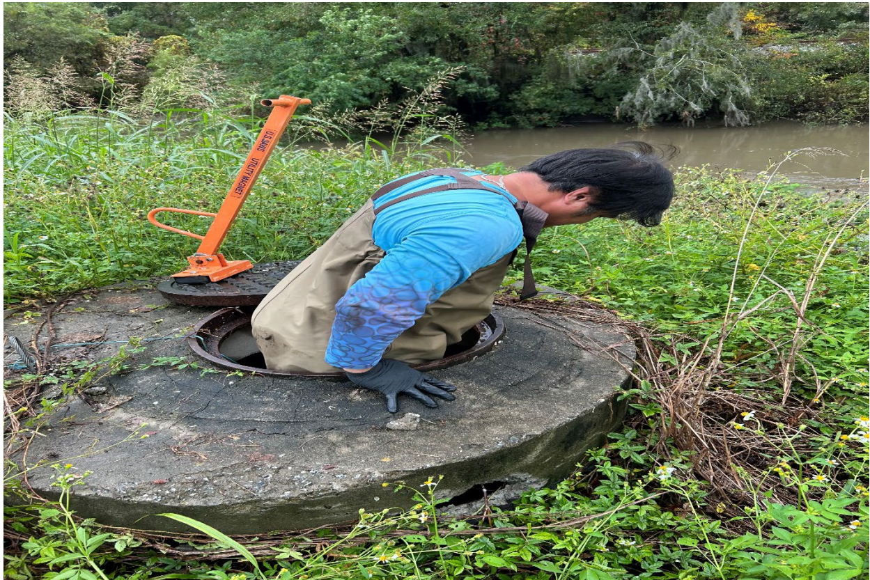
Releasing air for effluent lines. Pipe Makers Canal September 27
