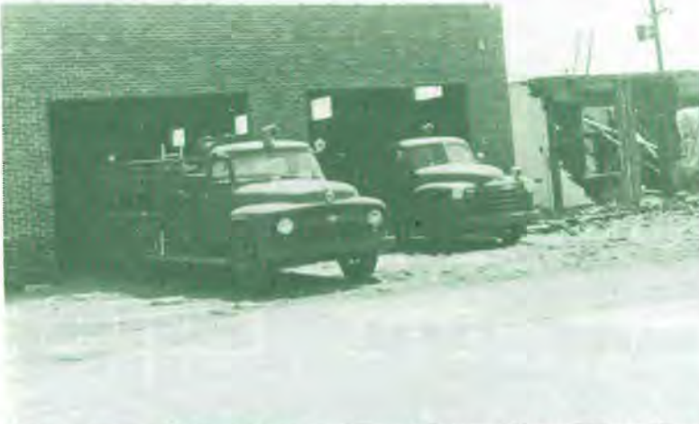
Construction of Garden City Fire Station
